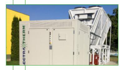
Geothermal Brine Power Output: 50 kWe
