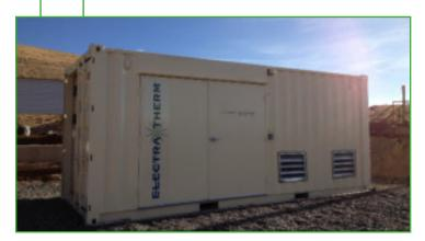
Geothermal Brine - Mining Power Output: 55 kWe
