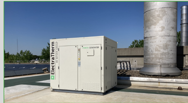
Waste Water Treatment Plant / Staten Island, NY
